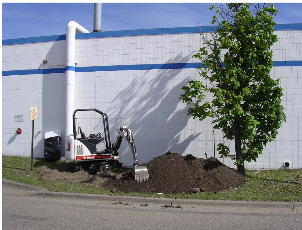
Figure 1. Excavation of insulation samples after 15 years
