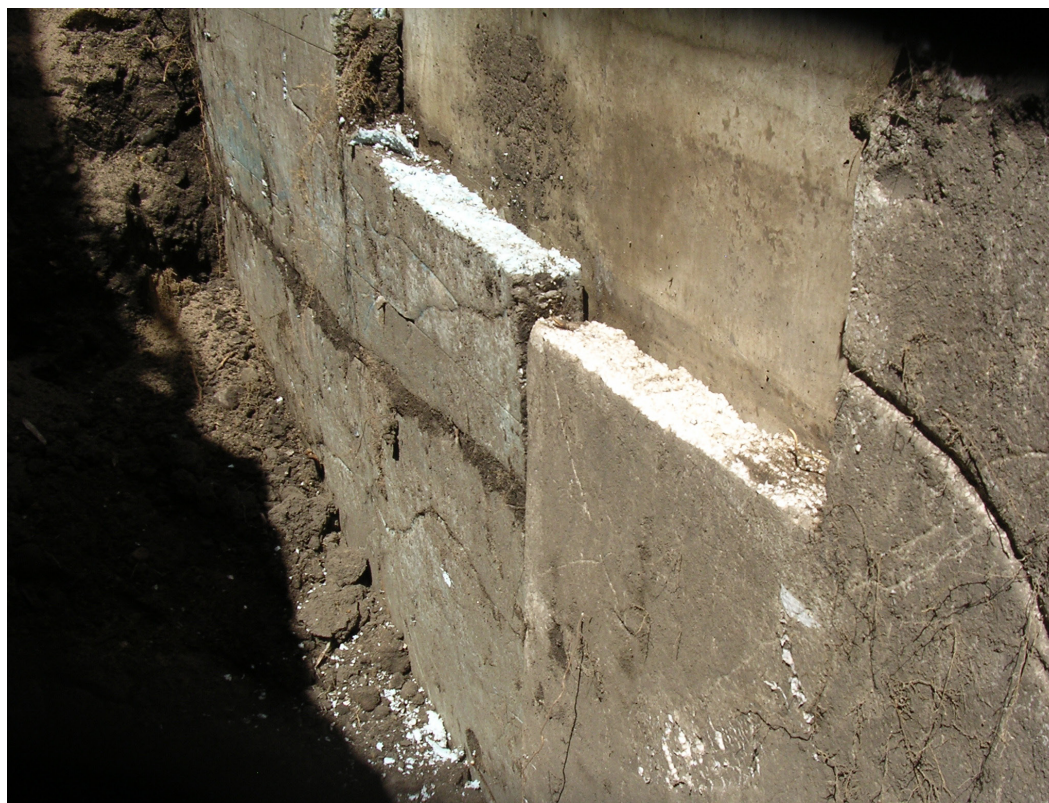
Figure 2. XPS and molded polystyrene below grade insulation
