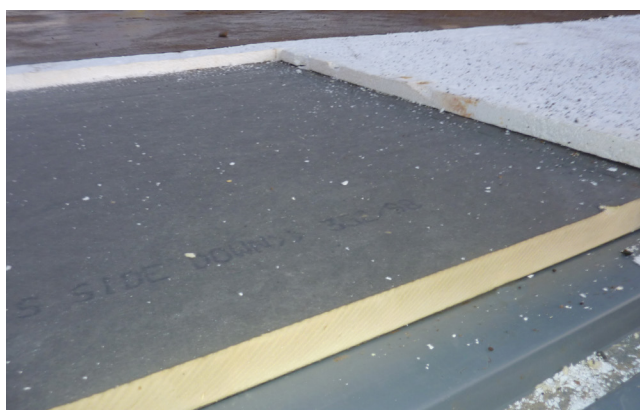
Figure 3. Existing roof being removed
